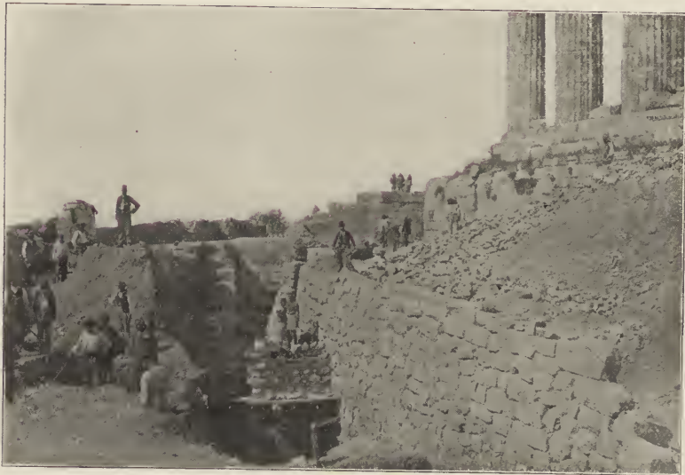
FIG. 29.—Foundation Walls of Parthenon on south side.
